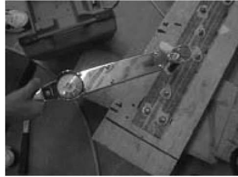
Fig. 7. Beam strengthened with mechanically fastened CFRP precured laminate
