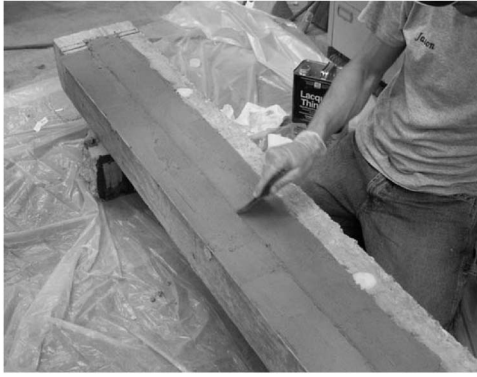
Fig. 6. Beam strengthened with bonded CFRP precured laminate (epoxy application)
