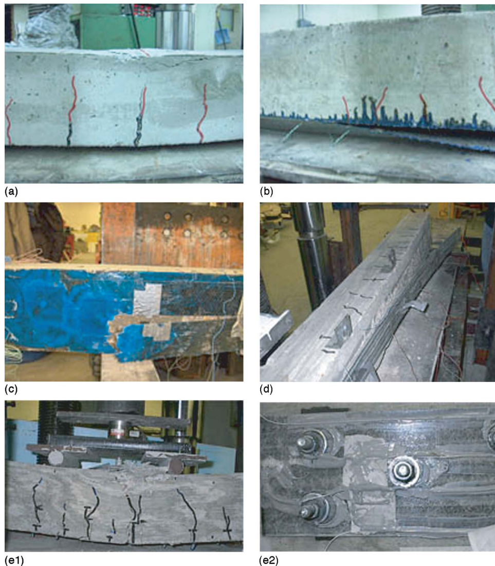
Fig. 13. Modes of failure of the specimens: (a) Unstrengthened control sample; (b) CFRP fabric; (c) CFRP fabric with anchor spikes; (d) bonded FRP precured laminate (bonded SafStrip); (e) MF-FRP system (bolted SafStrip)
