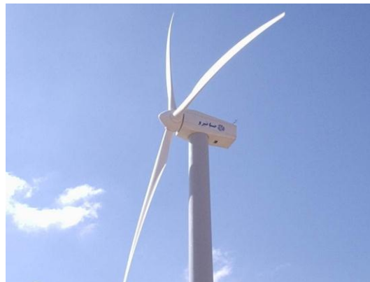
Fig. 2 Investigated 660 kW wind turbine (Courtesy of Sabaniroo Co., Iran)
