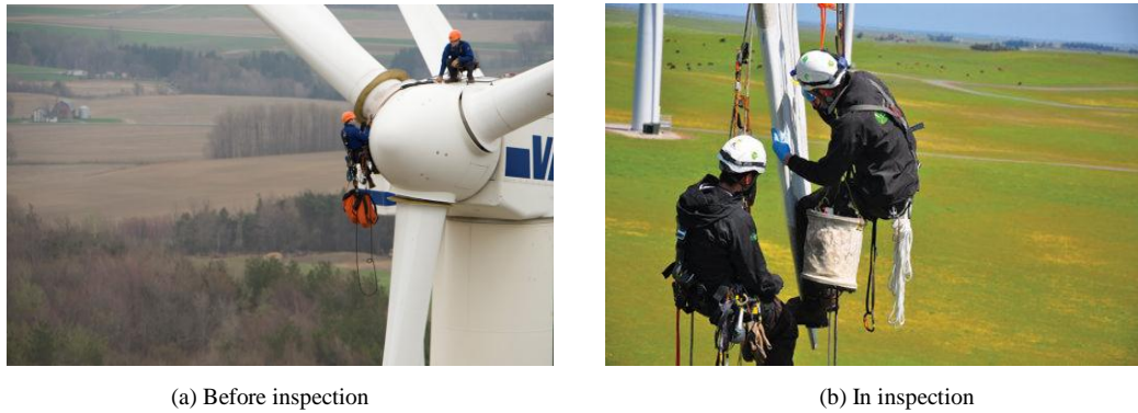
Fig. 21 Visual inspection of wind turbine blades
