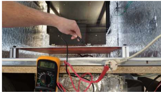
Fig. 129. Checking proper grounding.
