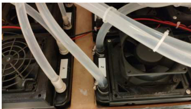
Fig. 103. Tubes installed on radiators.
