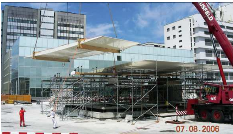
Fig. 1.6 Roof assembly at construction site
