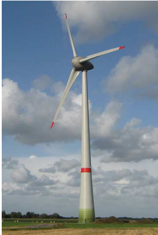
Fig. 1.3 7.5 MW Enercon E126 wind turbine. Hub height 135m, rotor diameter 126m. (Photo by jfz, licensed under a Creative Commons Attribution 3.0)
