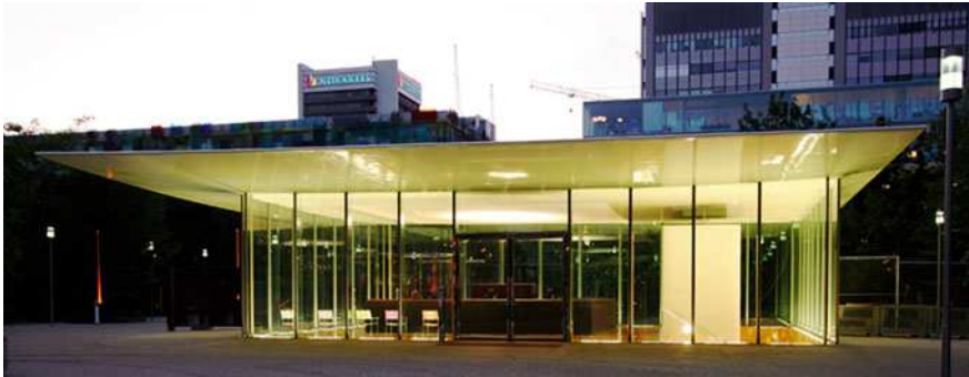
Fig. 1.5 Novartis Campus Main Gate Building with GFRP sandwich roof, view from the south
