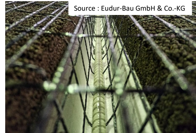
View into the element before concreting the load bearing structure
